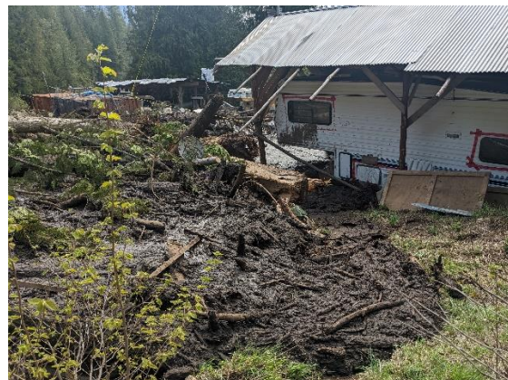
Photo 6. Debris flow deposit lobe adjacent to occupied dwelling at 3355 Little Slocan South Road
