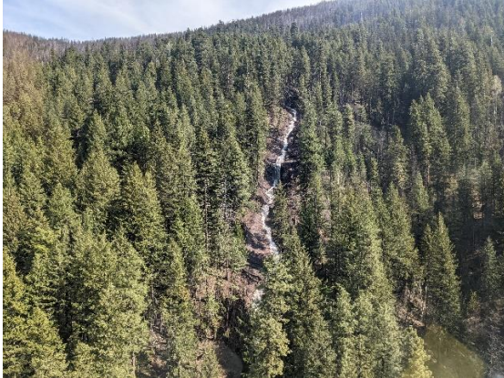
Photo 1. Debris flow path lower channel
