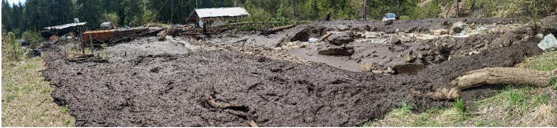
Photo 7. Debris flow deposit. Note lodged debris above and adjacent to the shipping container directing some flow down the driveway to the east and onto Little Slocan South Road.
